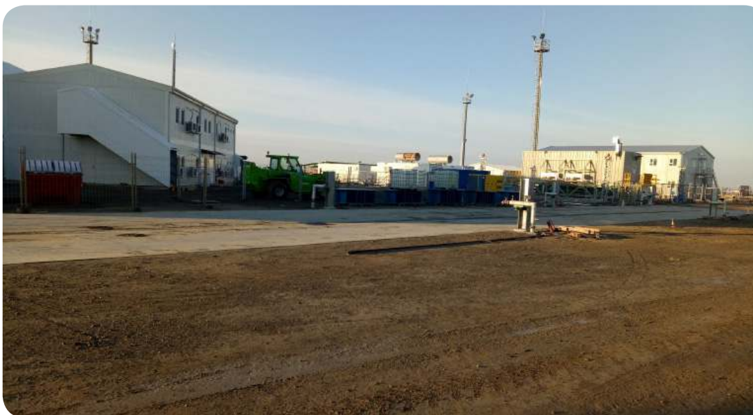
integrated washbay on the TCO project in CaTRo Kazakhstan
